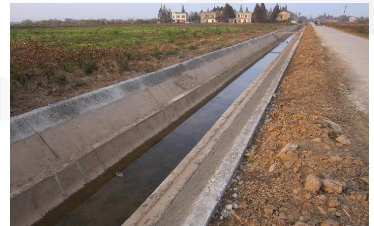
Canal Lining Concreted
