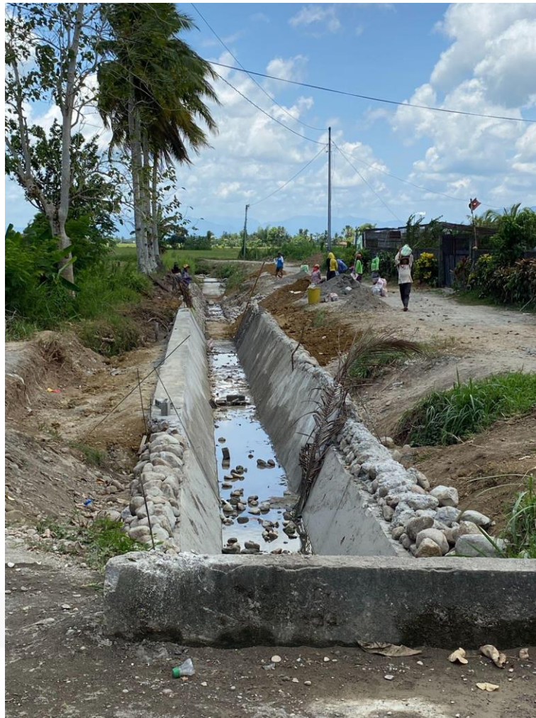
Target irrigation canal
