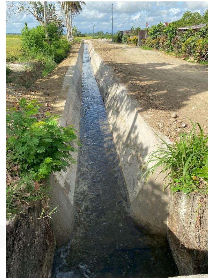
Target irrigation canal
