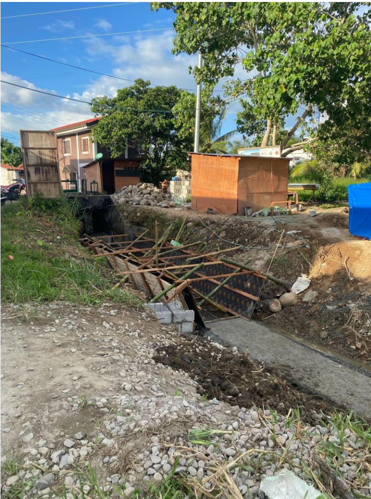
First 50 meters of the rehabilitation project
